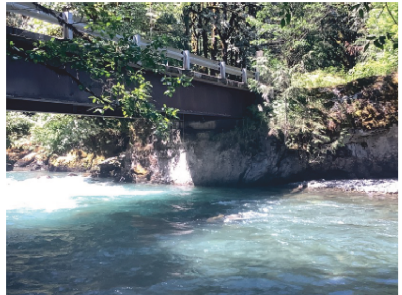
Left Bank Abutment when facing downstream
