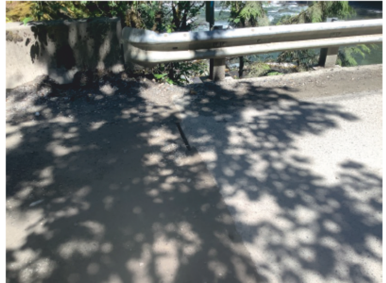
Deck joint between timber ballast walls
