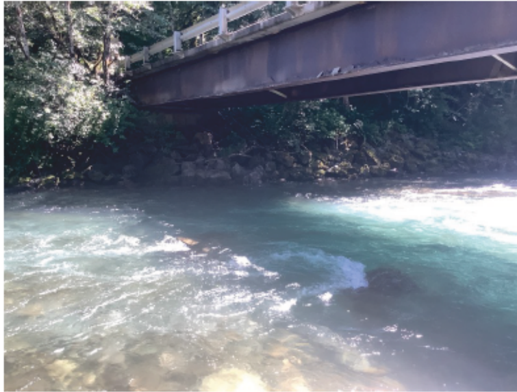
Right Bank Abutment when facing downstream
